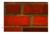
Mortar is harder, waterproof, less shrinkage, better bonding, more durable.
